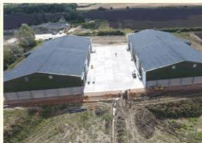
2016 Installation - two new 6000t flat stores with stirrers and automatic drying along with steel doorway barriers and a new weighbridge
