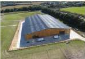
2015 Installation - greenfield site building of a new 73.2m by 45m cattle shed with the ability to be used for other showground activities
