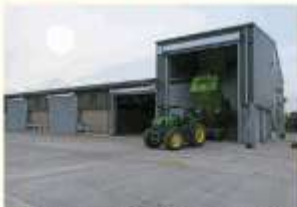
2017 Installation - conversion of existing cattle shed to grain storage and a new machinery bay inclusive of all new 100tph grain handling kit and a 34tph drier
